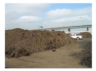
The second shift deposits un-amended Bio-Solid cake in similar rows to be left undisturbed for a period of 7 days. This material is then moved to a central collection site for removal to land application areas.
